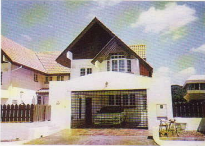
Remote-controlled garage door-cum-front gate.
